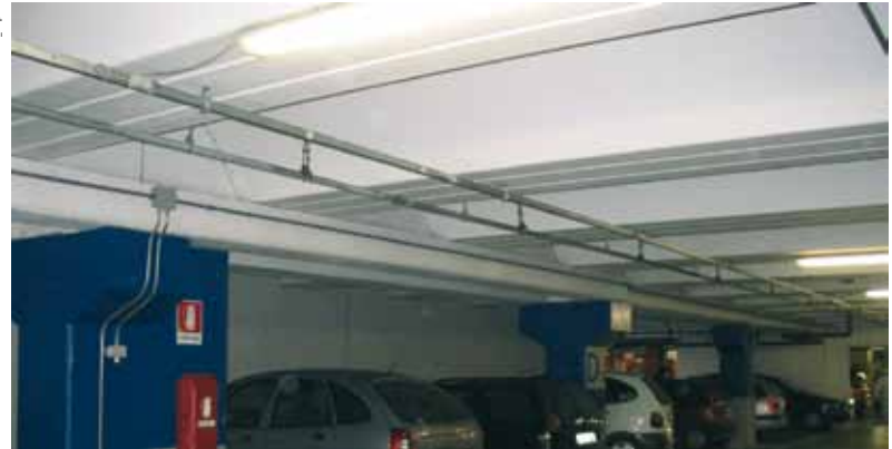
Canalis KBA supplying luminaires nearby sprinklers.
